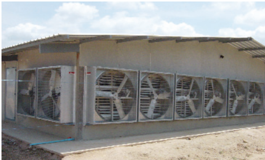
Figure 19: An Example of Power Ventilation
